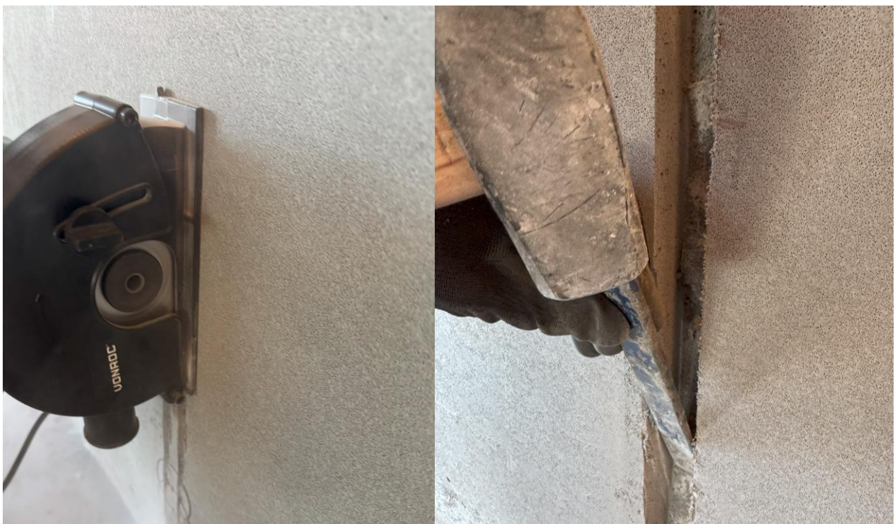
Wall chasers and chisels are used to create ducts for water and electric pipes.
